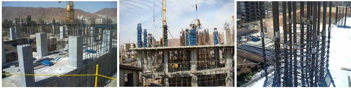
(a) Cast in place construction
