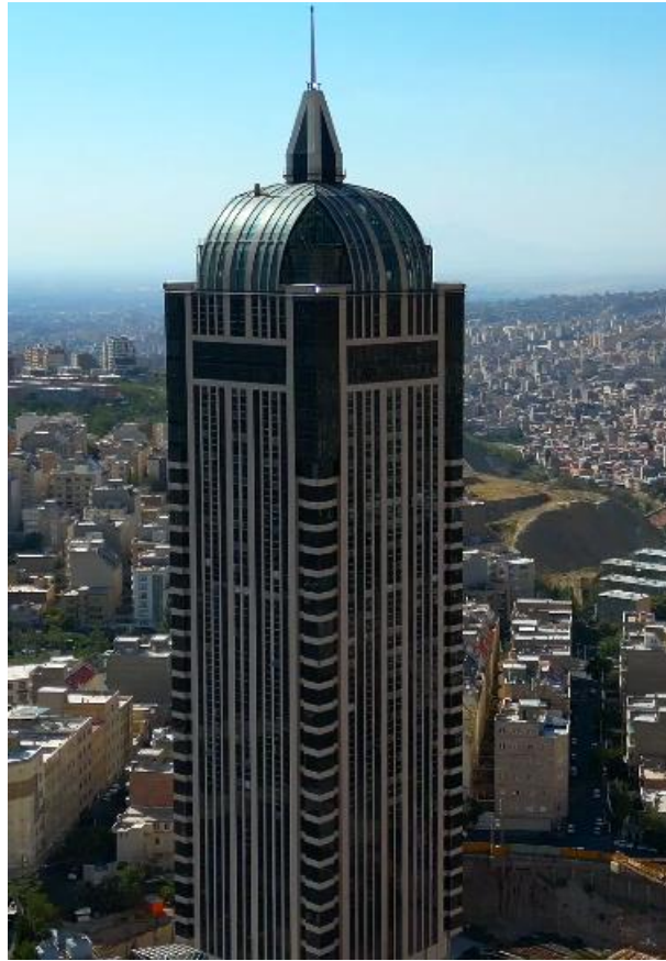
Figure 3- Overview of the World Trade Center Tabriz Building
