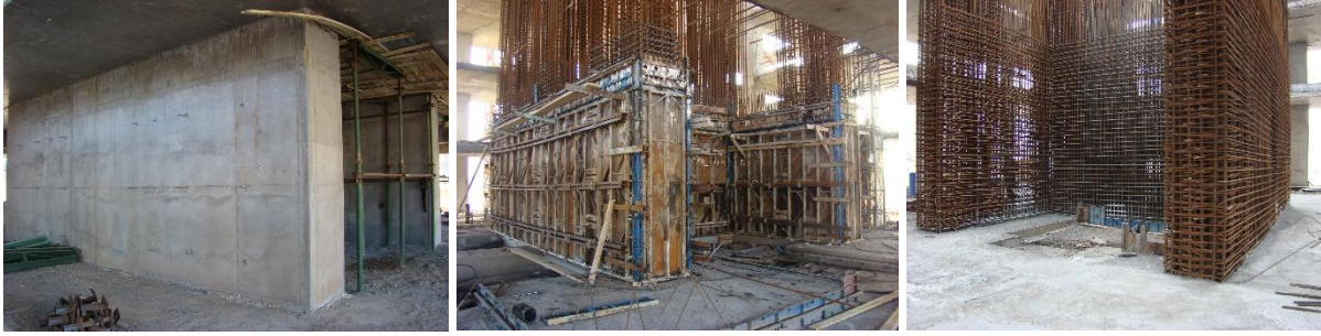
Figure 6- Photos of super wall implementation in Tabriz WTC building
