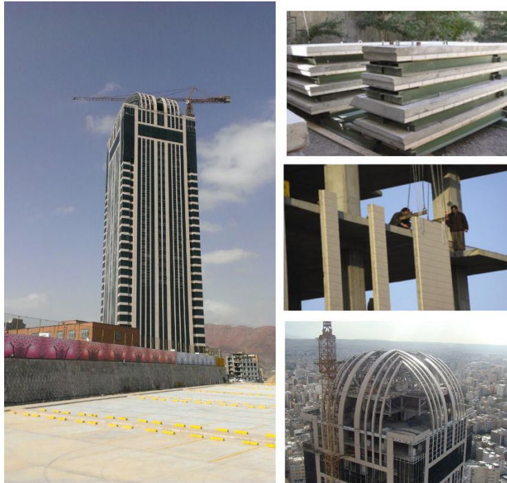
Figure 9- Photos of prefabricated facing panels in WTC Tabriz building
