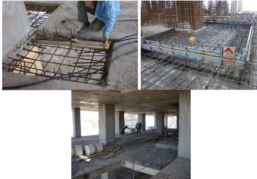
Figure 7- Photos of flat roof construction in WTC Tabriz building
