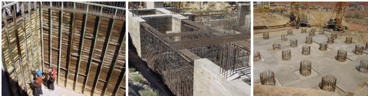
Figure 4- Photos of Cellular Raft Foundation constructed in WTC Tabriz.
